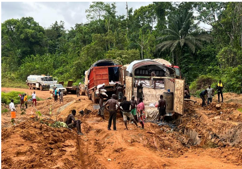
Figure 19: Road conditions worsening, especially in the South East
